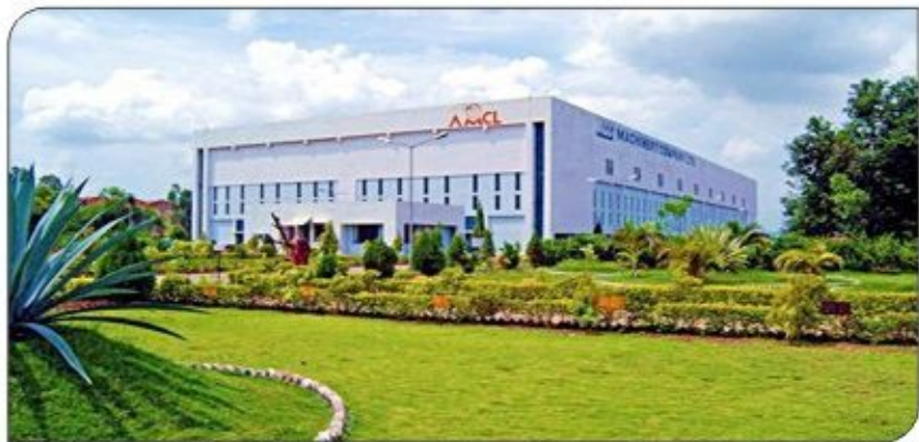
Works at Nagpur
